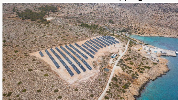
Halki Solar Park. Photo: ChalkiON project
